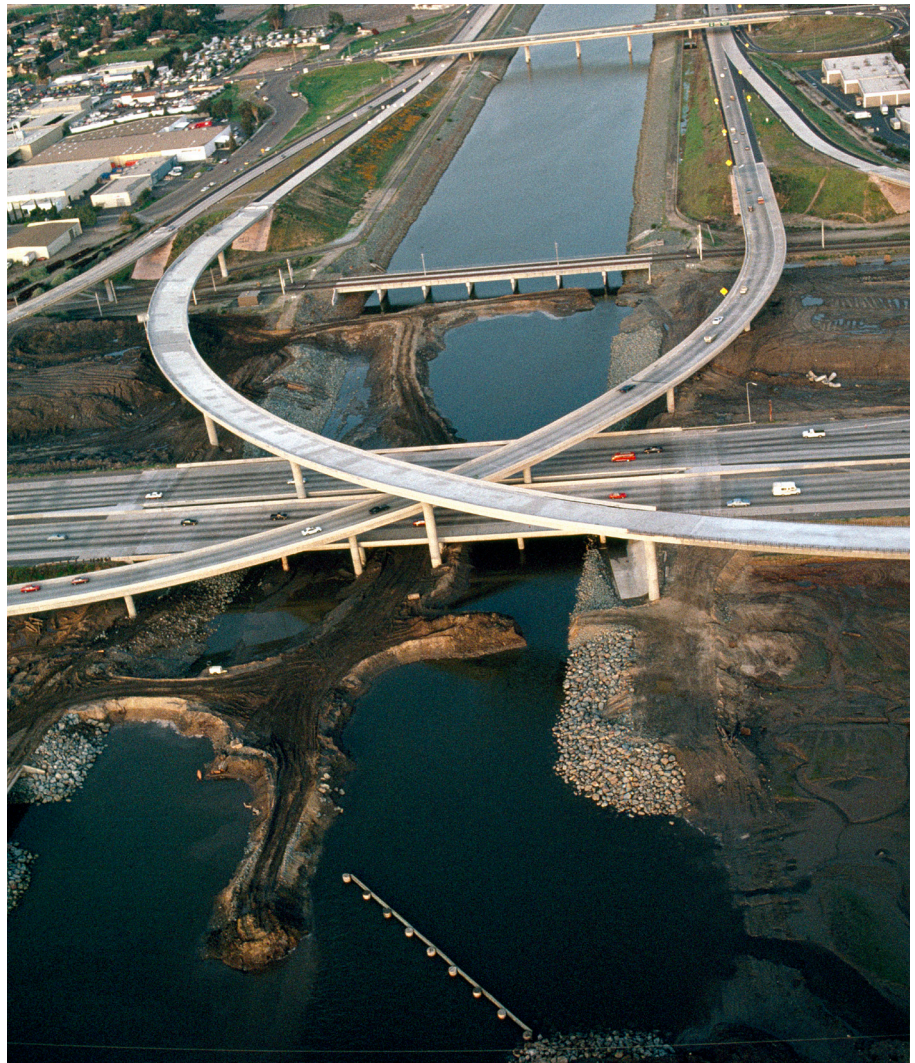
Roads over Sweetwater Marsh, San Diego, California
